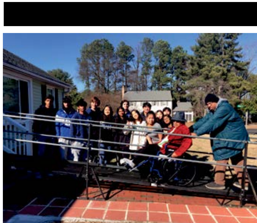
Students from Deep Run High School stand behind the ramp they just built for Thelma, a Henrico County Resident with multiple health problems.
